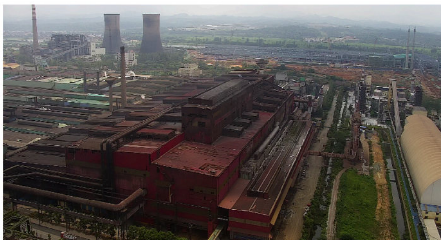
钢一区转炉炼钢厂房顶已无烟气外溢现象
