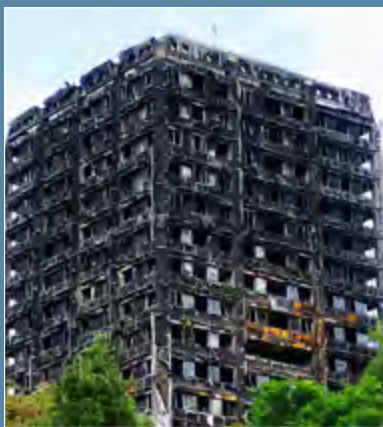
Grenfell Tower following the 2017 fire. Photo credit: Alex Donohue | iStock
