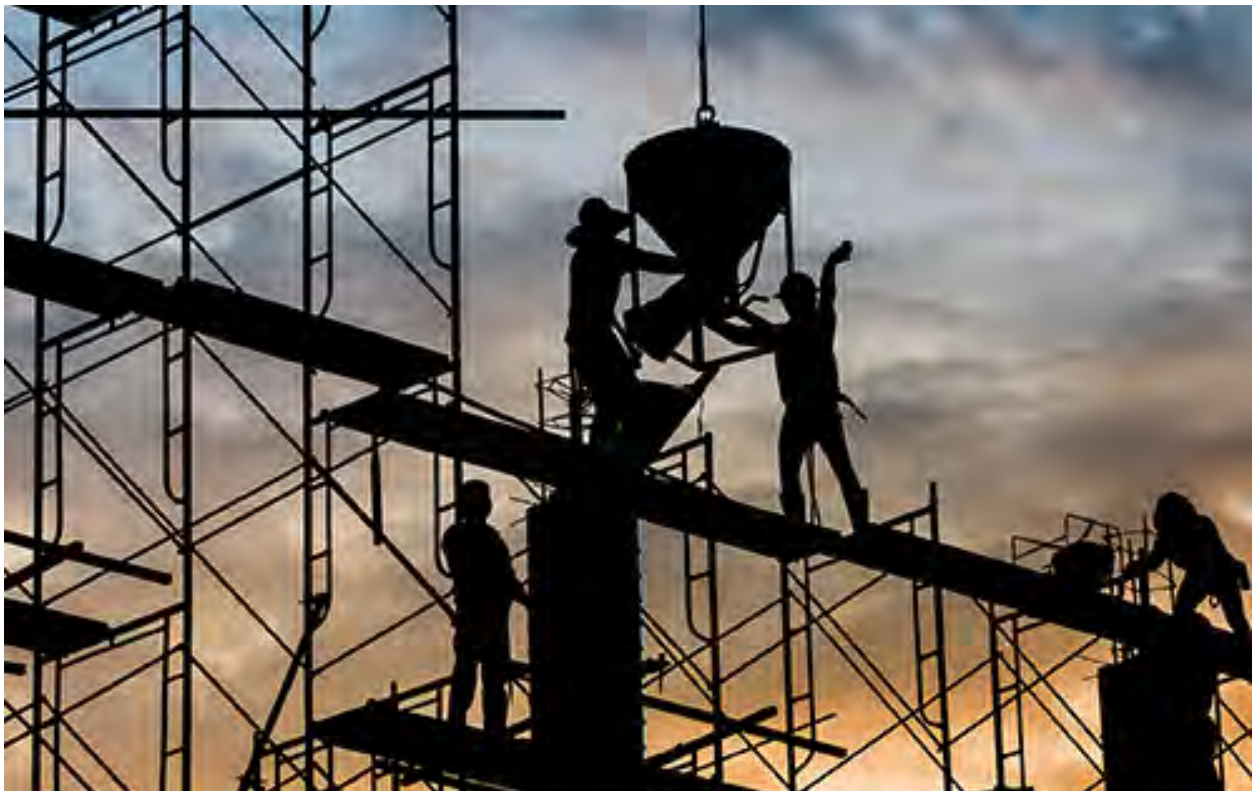
Figure 11.3 // Construction workers casting concrete on site
