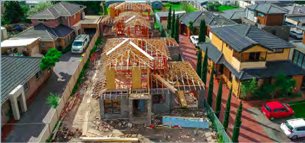
Building construction in Melbourne, Australia. Photo credit: Elias Bitar | iStock
