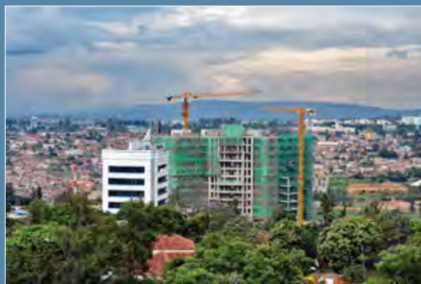
Building construction in Kigali. Photo credit: Sloop | iStock
