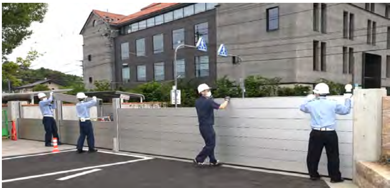
Figure 7.3 // Temporary flood gates being installed at the Kurashiki Central Hospital in Japan as part of a dry flood-proofing strategy
