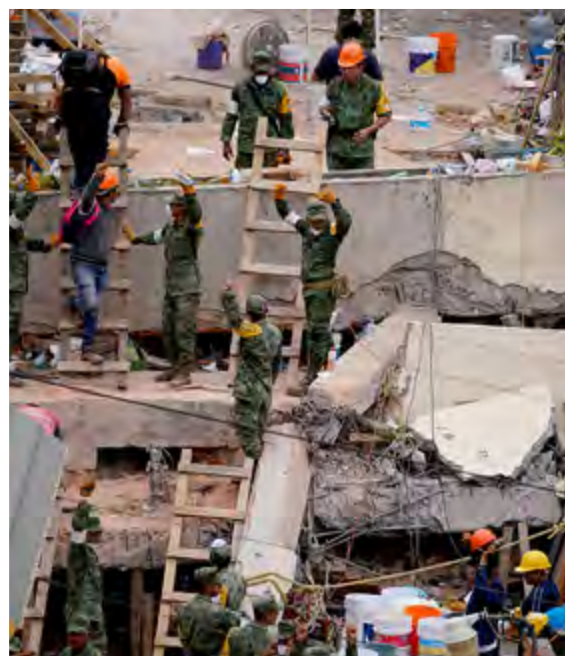
Figure 4.5 // Rescue efforts after the collapse of the Enrique Rebsamen School, Mexico City in the 2017 Puebla earthquake.
