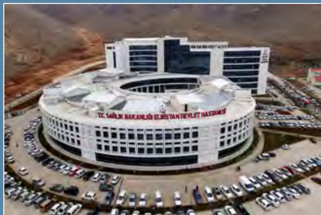
Seismically Isolated Elbistan State Hospital in Türkiye (Qu, 2023)
