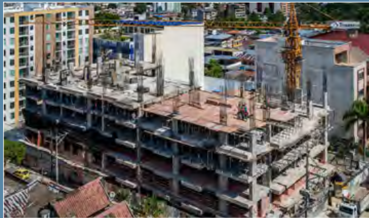
Building construction in Colombia. Photo credit: Giorgio Morara | iStock
