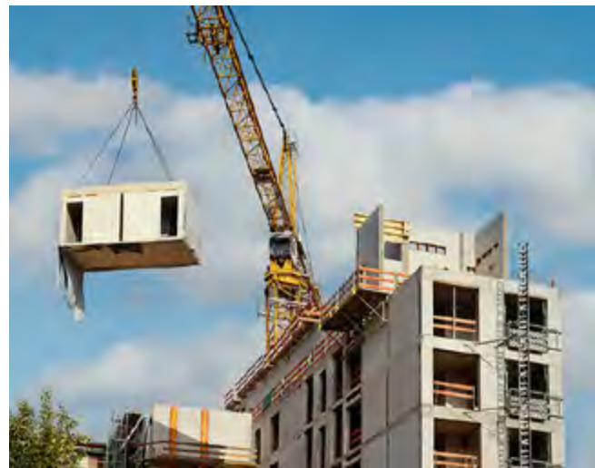
Figure 9.2 // Construction of modular mass timber building
