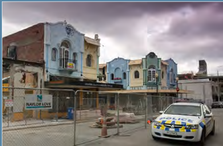
Cordoned-off buildings in Christchurch, New Zealand. Photo credit: Kokkai Ng | iStock
